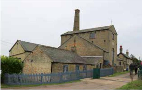
*The imposing buildings of Stretham Pumping Station. The engine is in the tall building while the scoop wheel it drives is in the one this side of it.*
