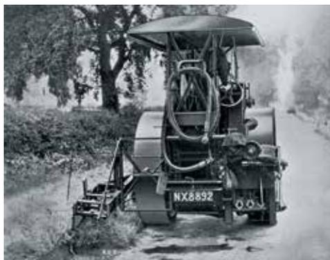
*The Patent Excavator in use cutting below road level behind Aveling & Porter 10 ton piston valve compound roller No. 11254 of June 1925 (NX 8892), supplied new to Warwickshire C.C., becoming their fleet No.9.*
