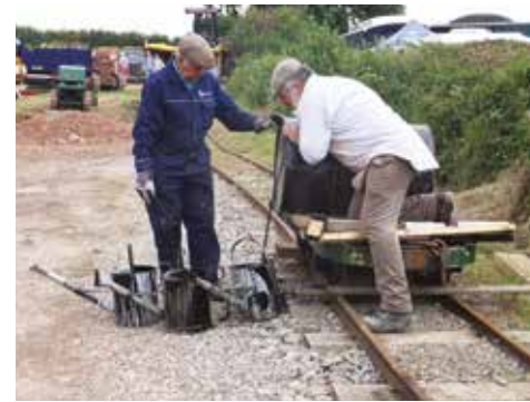
Pouring the tar into can.
