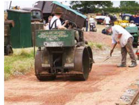
Spreading the chippings for rolling.
