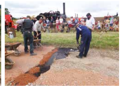
Applying the tar.
