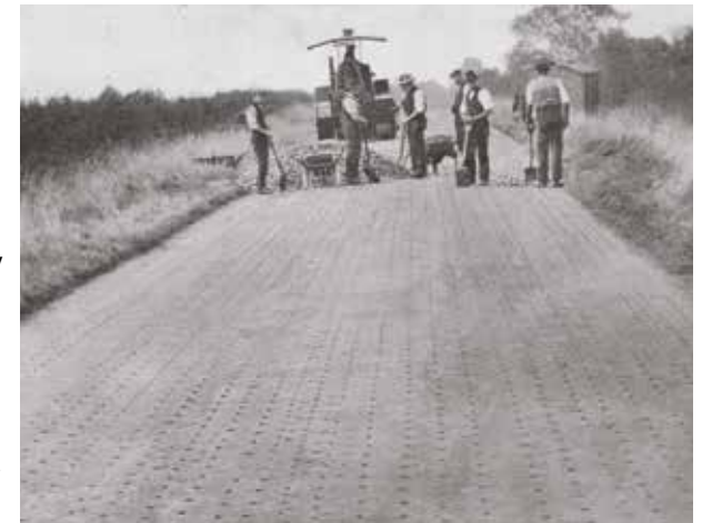
The Aveling Road Indenter in use when fitted to one of their piston valve rollers. This was Aveling 10 ton single No.11250 of June 1923 owned by Bedfordshire County Council, their fleet No.2.
