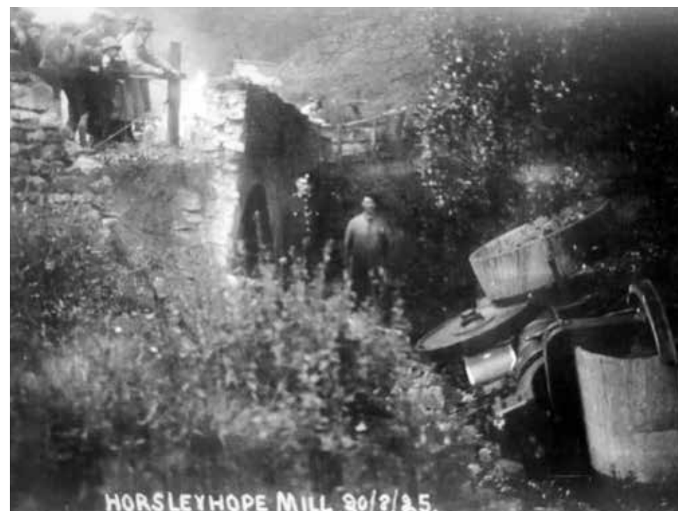
Another view, taken from further down, showing the roller on its side at the bottom of the banking.
