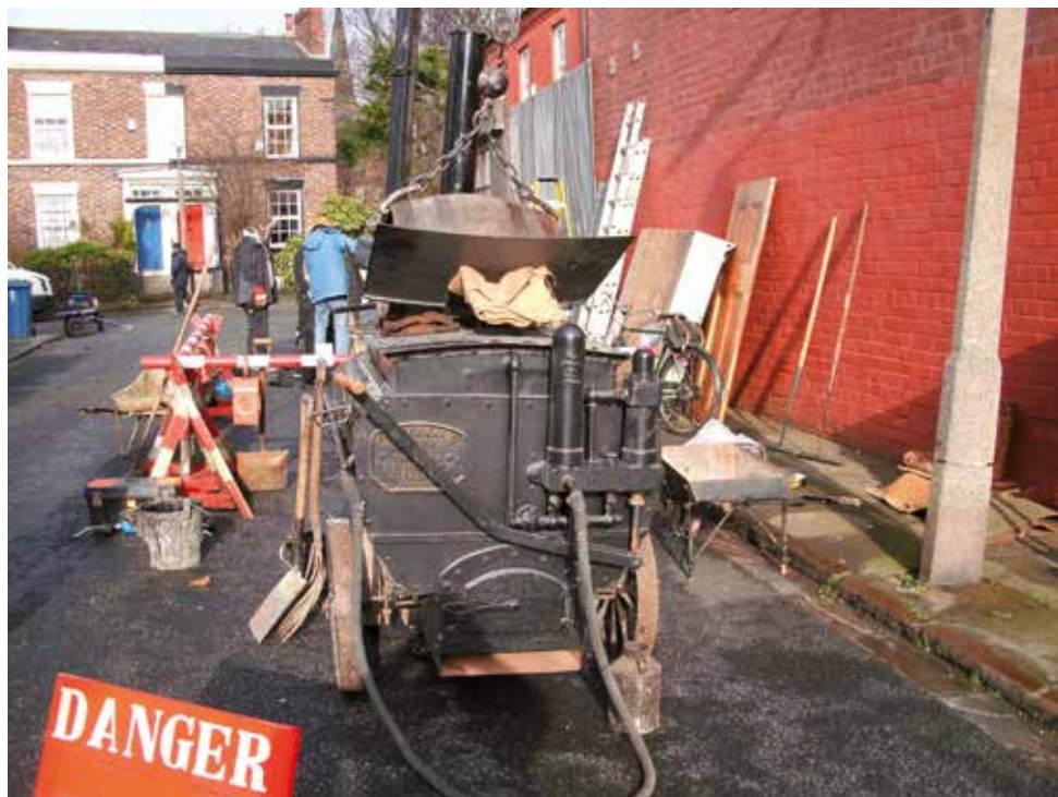
The tar boiler in all its glory on a Liverpool street.
