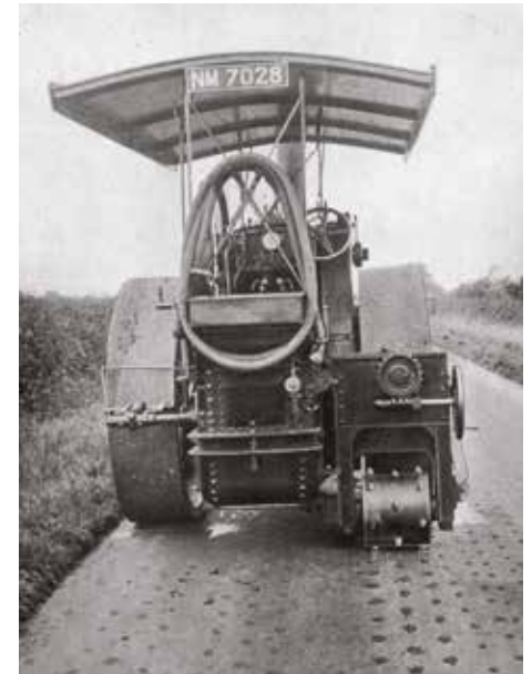
The Aveling Road Indenter in use when fitted to one of their piston valve rollers. This was Aveling 10 ton single No.11250 of June 1923 owned by Bedfordshire County Council, their fleet No.2.
