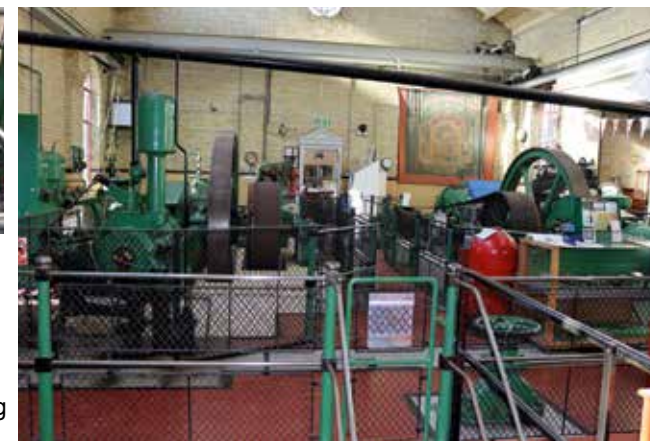
A general view of the two Campbell oil engines in the Old Brook Pumping Station. The pumps are at the far end.
