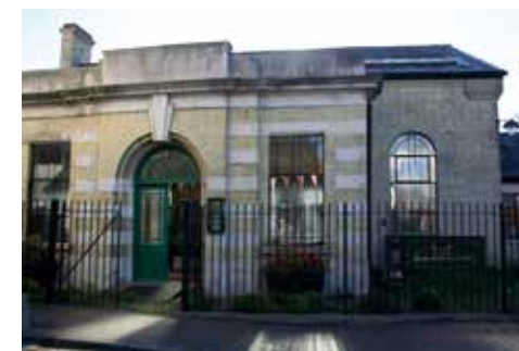
The front of the Old Brook Pumping Station in Chatham.
