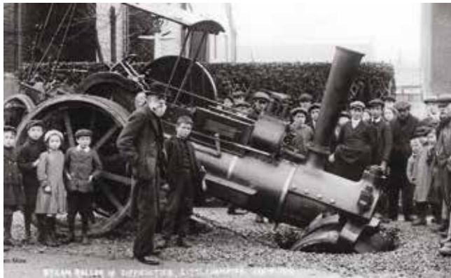
At Littlehampton, in January 1914, the front end of the Wallis & Steevens roller is well down into the cavity in the roadway.
