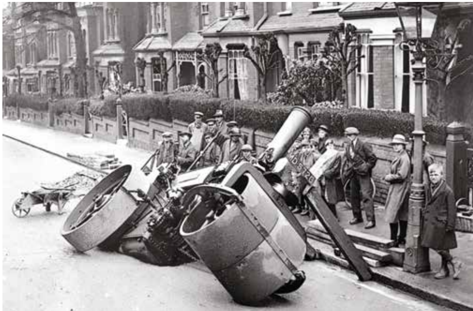
This accident, involving an Aveling roller ten years later in Highgate, London, in April 1924, inevitably attracted the usual group of interested bystanders. It can be seen that someone has had the foresight of propping the roller up on its left hand side with a baulk of timber so that it doesn't fall over any further.
