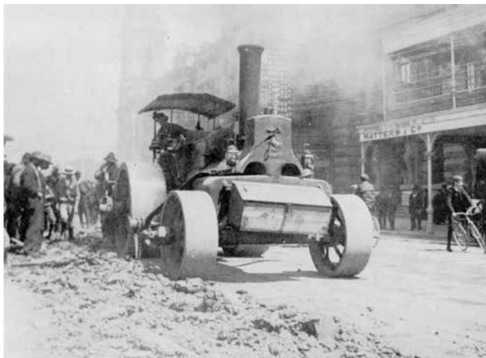
The roller is using its scarifier to loosen the existing top surface of the road in order to eventually prepare a suitable base for the new tram tracks.
